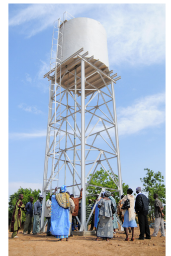
Elevated storage tanks, like the one shown here, help to bring water to a broad network of water access points.
