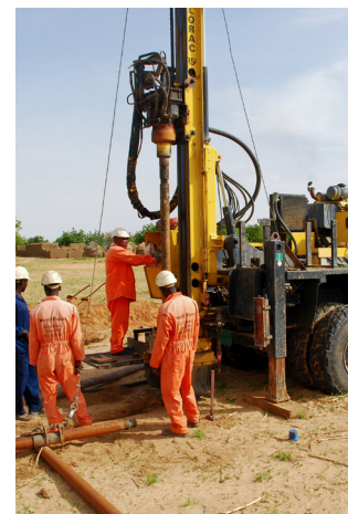
World Vision workers operate a portable drilling rig. Deep wells can be drilled to hundreds of feet to provide consistent water all year.
